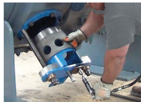
Drill moving assembly into valve port
